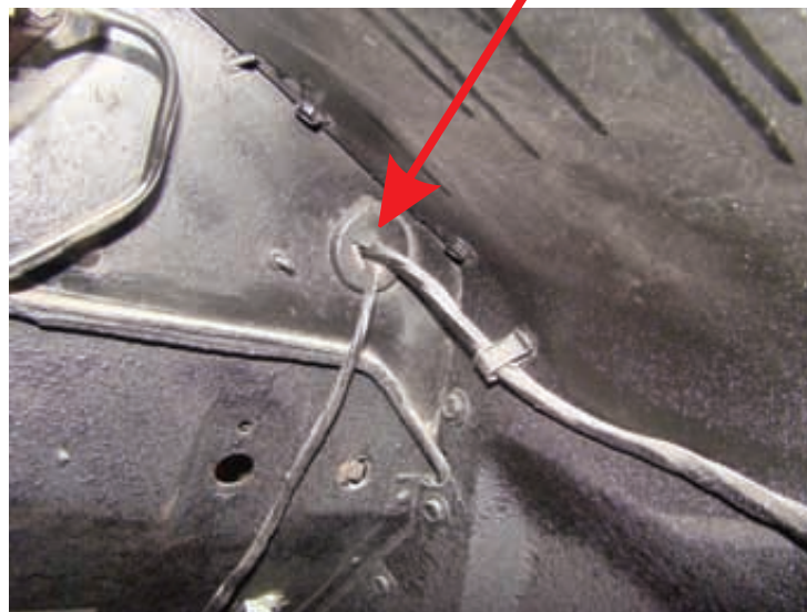
Front Light Wiring
